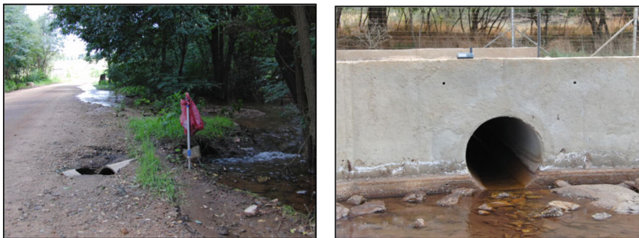
Plate 9 Original SDM flow gauging station MRd in separated pipe (below left, 05/02/2010) and one of two identical replacement culverts (below right, 05/10/2010) beneath the reconstructed gravel Malmani Road across the Riet Spruit at this location
