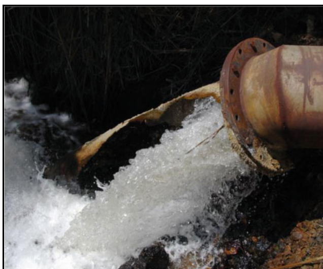
Plate 1 Corrosion of large-diameter pipe draining the Aviary Dam on the Tweelopie Spruit in the KGR; photo at left shows remnant (at bottom centre) tenuously attached to flange, and photo at right shows close-up view from opposite side
