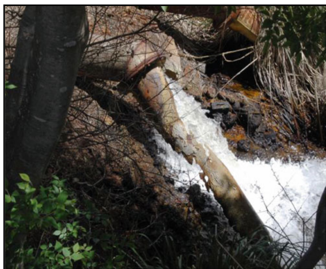
Plate 1 Corrosion of large-diameter pipe draining the Aviary Dam on the Tweelopie Spruit in the KGR; photo at left shows remnant (at bottom centre) tenuously attached to flange, and photo at right shows close-up view from opposite side
