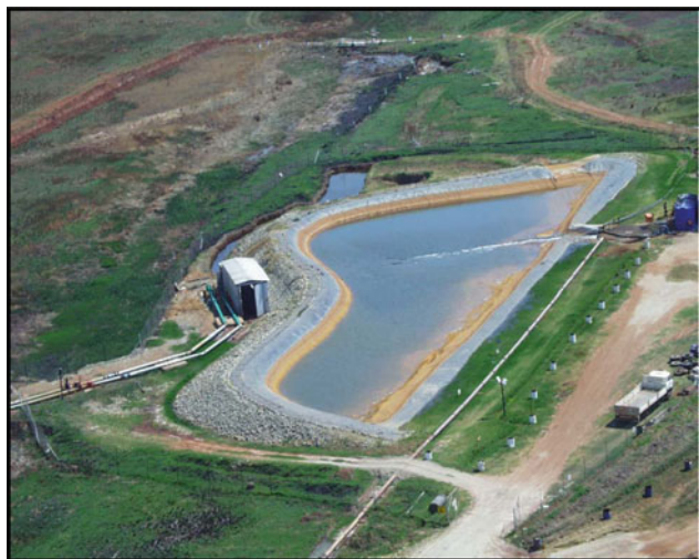
Plate 3 Aerial view (looking north) of the HDPE-lined off-channel storage dam shortly after construction at the Black Reef Incline (circular structure at centre right) to contain mine water decanting from this structure; also visible are the pump station (centre left), the gravity-fed pipeline (45° diagonal from centre bottom) draining the upstream in-channel Portuguese Dam, and the course of the Tweelapie Spruit exiting picture at centre top (photo G Krige, 05/10/2004)
