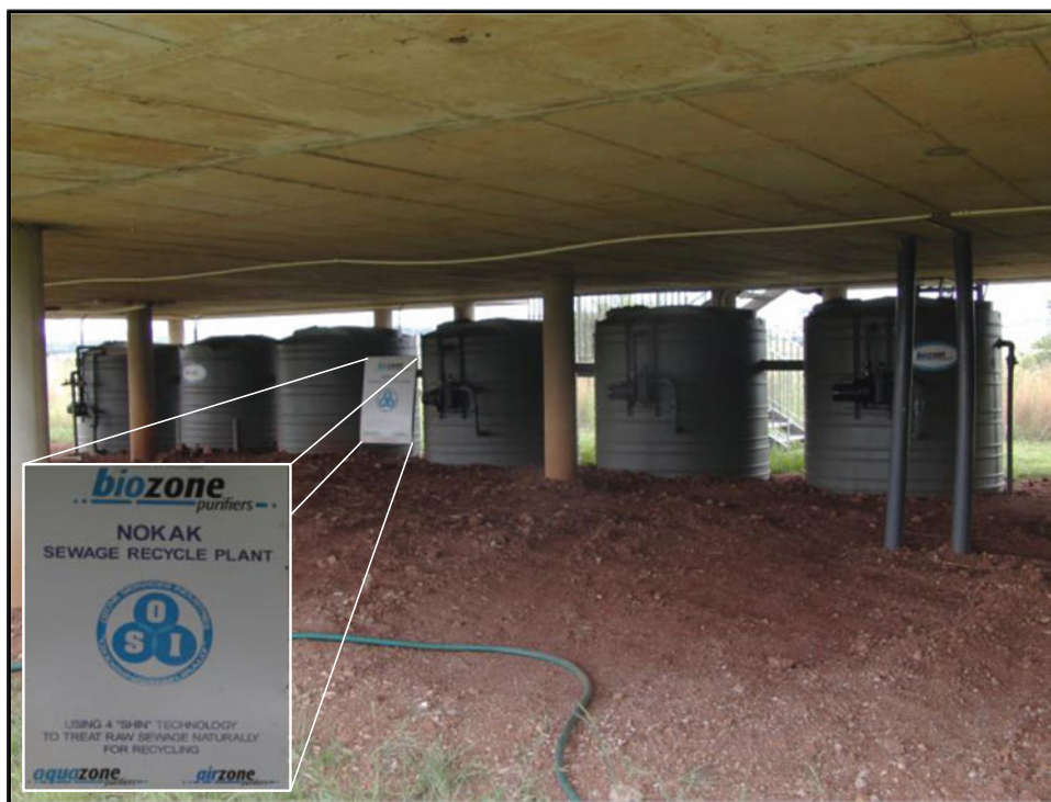
Plate 3 View of the biozone sewage treatment plant installed under the Sterkfontein Cave Visitor Center in mid-2011
