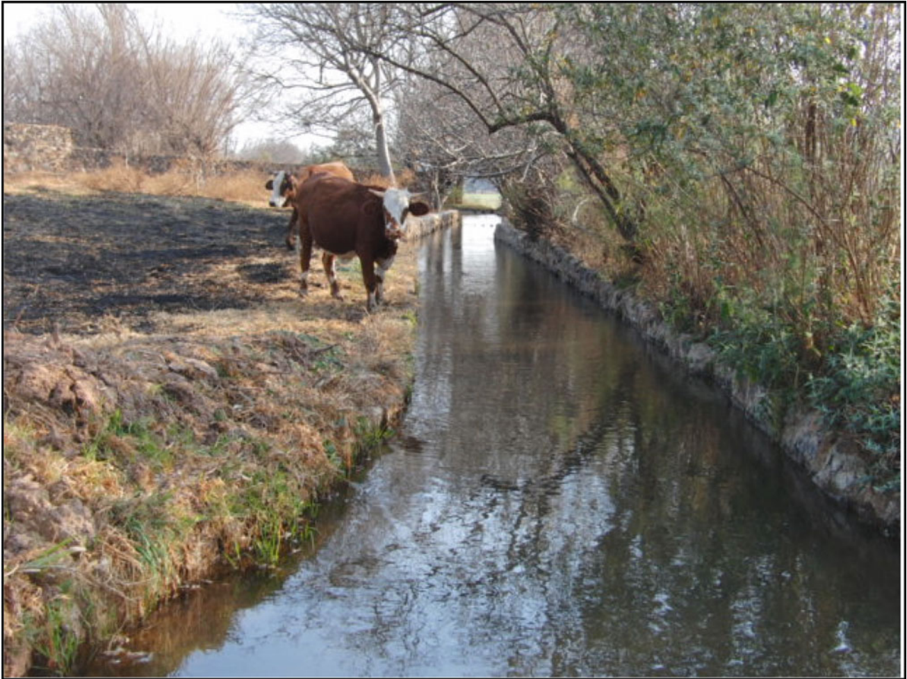
Plate 13 View of the ~100-year old A-furrow at Ptn 8 of Kromdraai 520JQ, looking upstream; flow measured at ~154 L/s on date of photo
