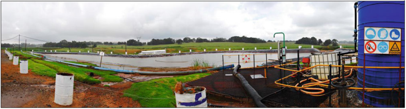
Plate 3 Panoramic view of the HDPE-lined dam at the Black Reef Incline (under grid at front right-of-centre), showing the pump station at left-of-centre beyond the dam, from where the water is pumped to the HDS treatment plant located on the skyline (continental divide) at left
