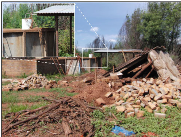
Plate 2 Damage to infrastructure caused in the upper reaches of the Skeerpoort River valley by a flash flood in October 2009; note flood stage height of \sim 2 m as indicated by the drift debris on pump house roof and in inset picture
