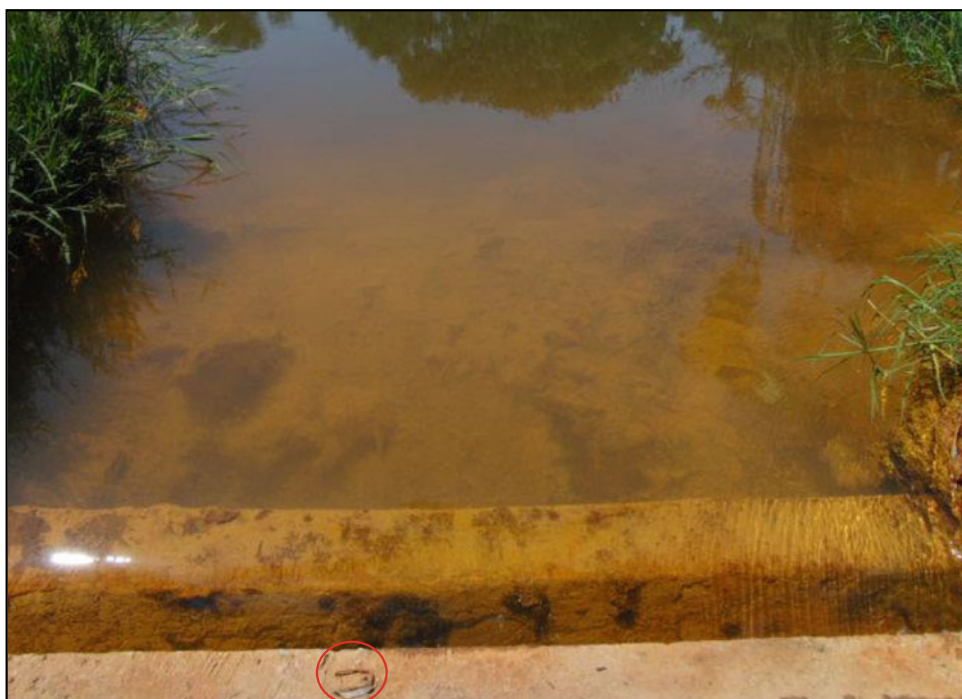
Plate 3 View of station F11S12 showing concrete weir coated with freshly precipitated hydrous ferric oxide or ferrihydrite ( 5\text{Fe}_2\text{O}_3 \cdot 9\text{H}_2\text{O} ) and object (circled) on causeway for common reference with Plate 2
