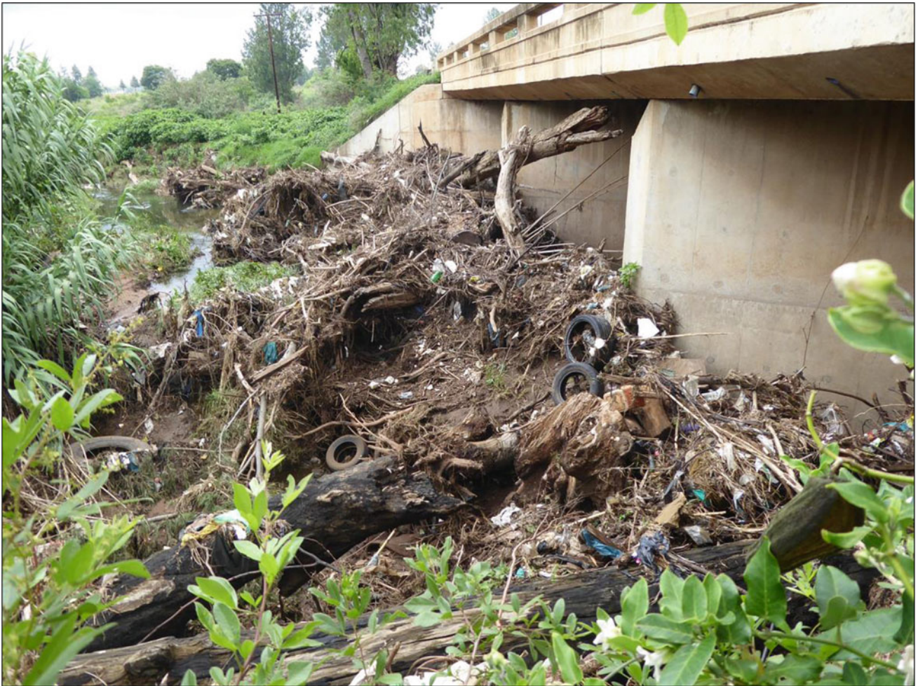
Accumulation of flood debris blocking the entrance to culverts of the N14 bridge over the Blougat Spruit near Oaktree; the hazard for potential flood damage to the national road is self-evident
