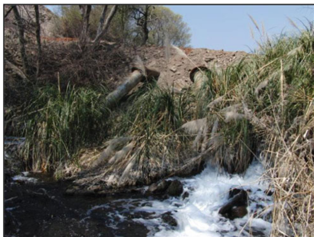
Plate 12 Overflow of the Aviary Dam (impounded by the earth embankment at rear of photo) at the northern end of the KGR; compare condition of outlet pipe at left with that of same pipe in Plate 1 in Chapter “Chemical Hydrology”
