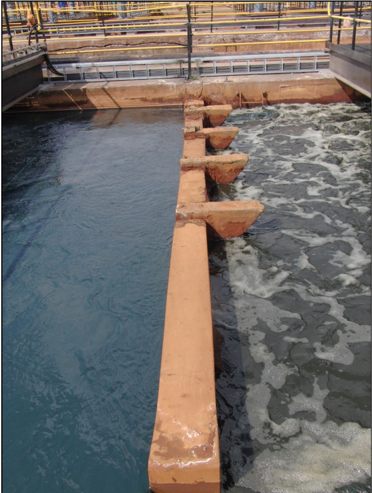
View of the first portion of the newly constructed and commissioned Train 4 (of 4) of the high density sludge (HDS) mine water treatment plant showing \text{CaCO}_3 -dosed raw mine water moving from stirred condition (left) to aerated condition (right); trains 3 to 1 extend to back of view (photo P Hobbs, date 11/05/2012)
